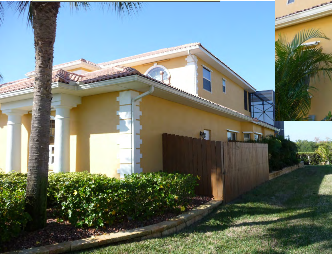
NE corner view
