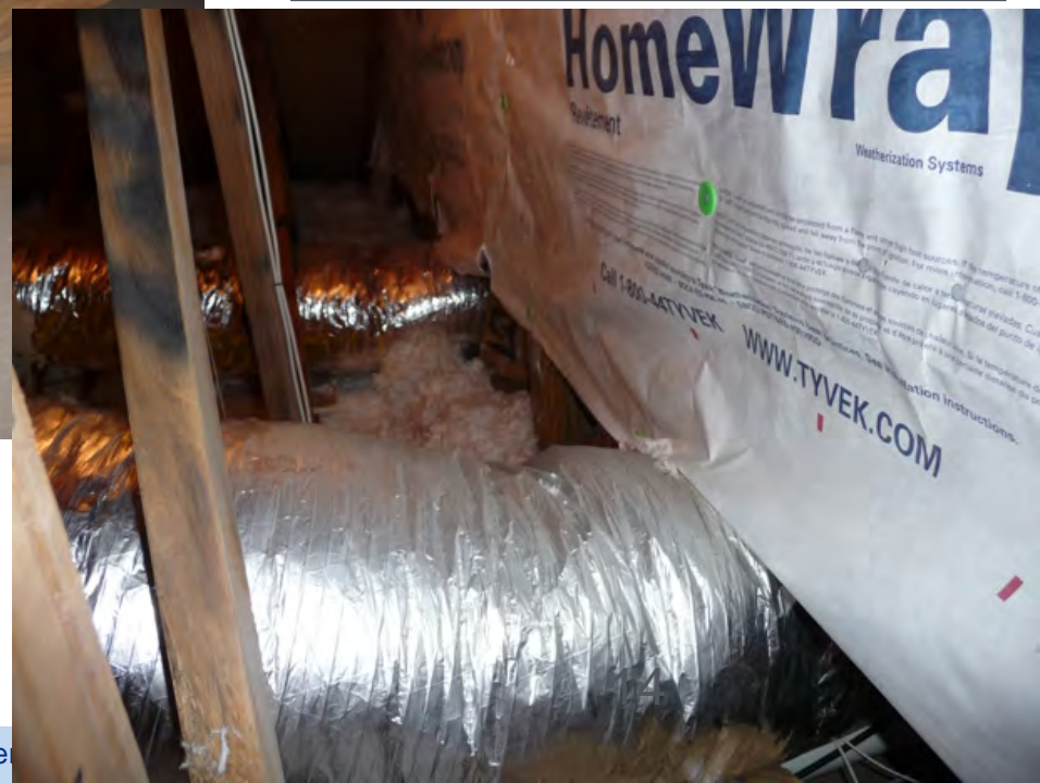
West side attic view
