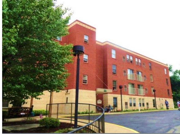
Multifamily buildings in Pennsylvania (Photo Courtesy ACTION Housing)
